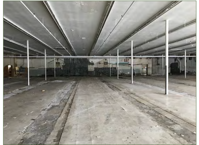
Figure 9 – Inside the Homer Avenue Plaza, the future host site for the year-round farmers market is mostly a blank slate. The YMCA currently owns the building, but hopes to convert it to a multi-purpose space with Seven Valleys Health Coalition and other partners. Image credit: Northbound Ventures
