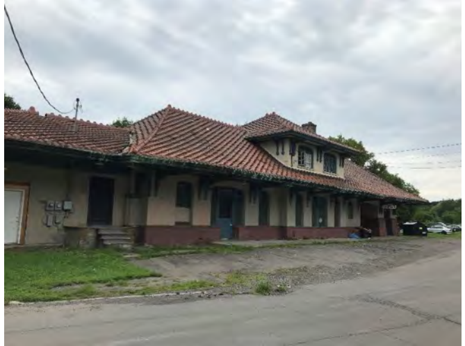
Figure 8 – The old rail passenger depot is a redevelopment opportunity in the heart of the city.
