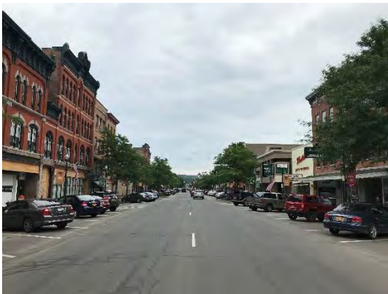
Figure 2 - Cortland is looking to convert its Main Street from one-way to two-way in order to calm traffic and encourage economic development. Image credit: EPR
